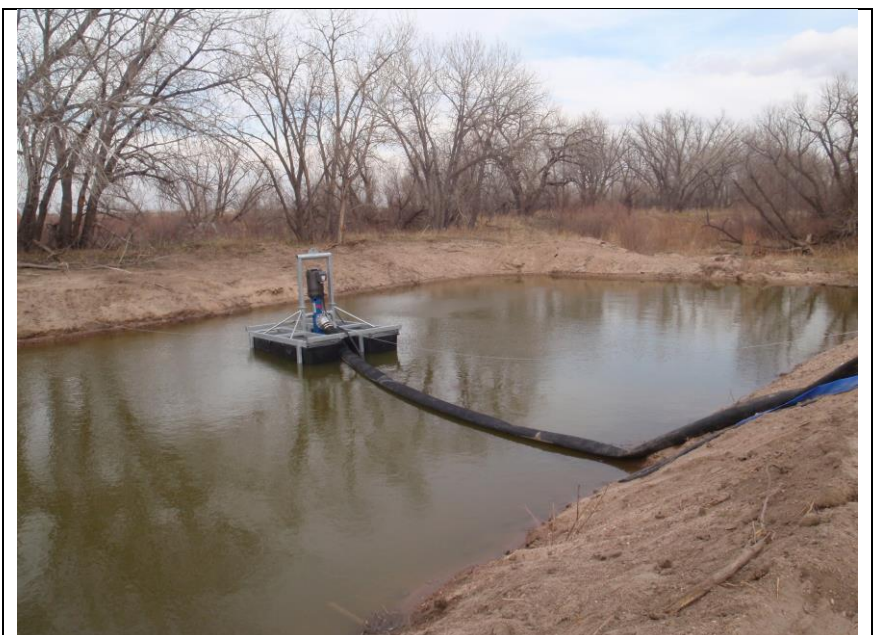
Figure 5. Heyborne Lift Station
